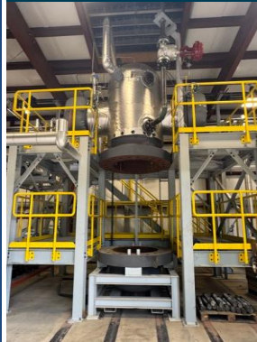
5 Vibration Systems installed
