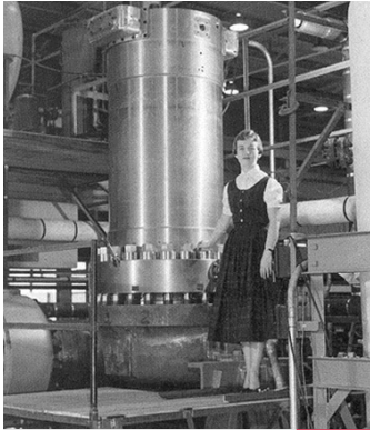
Reactor Coolant Pump Shippingport PA
