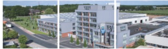
Zeven, Germany – Main plant
